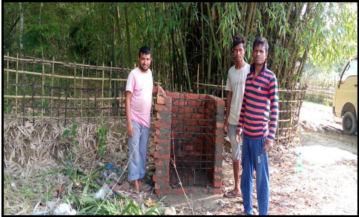
Photo: Construction of Dustbin under Green and Clean Campaign of College, 20-05-2022
