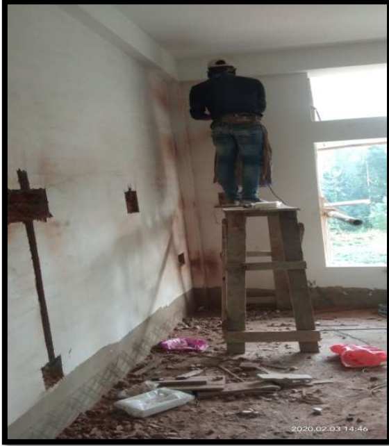
Fig. Mr. Anshuman Bora, Professional Electrician (Batch: 2017-2019) while doing Domestic Conceal Wiring
