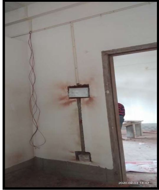
Fig. Mr. Anshuman Bora, Professional Electrician (Batch: 2017-2019) while doing Domestic Conceal Wiring
