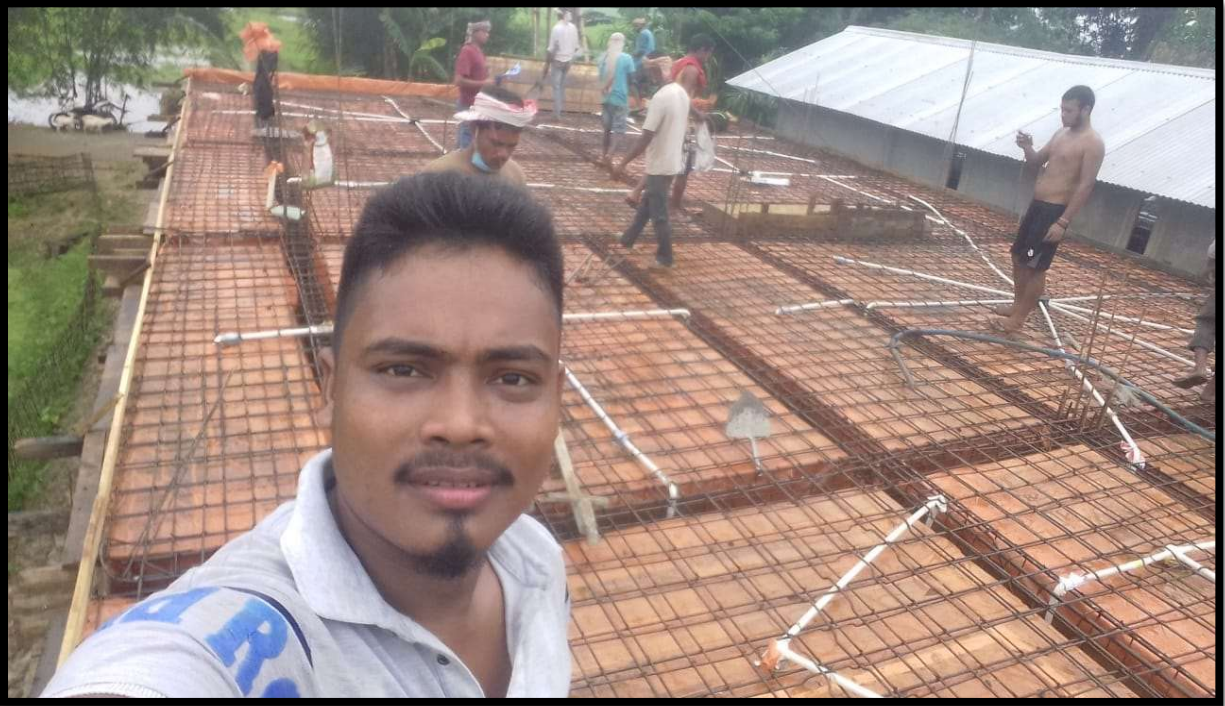
Fig. Mr. Pranjal Saikia and his Group (Batch: 2017-19) while doing Conceal House wiring
